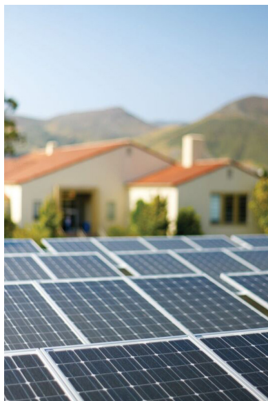
Solar panels atop Building 21
